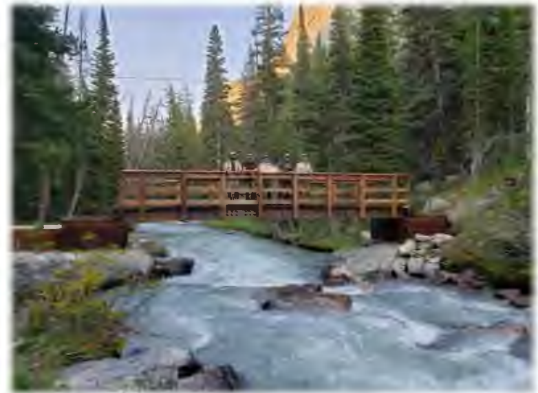
Shoshone – Downs Fork Trail Bridge (FLTP/GAOA LRF Project)
