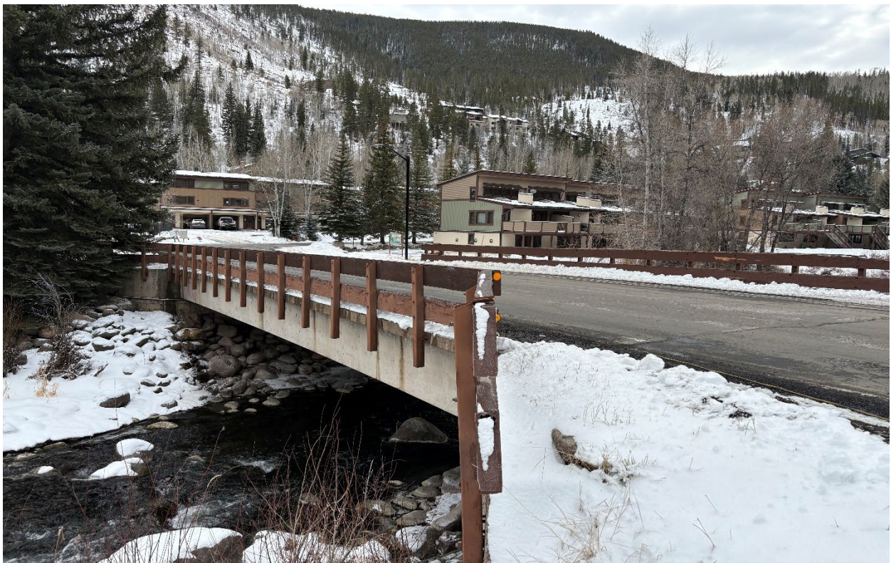
East side of the east Kinnickinnick Bridge looking south
