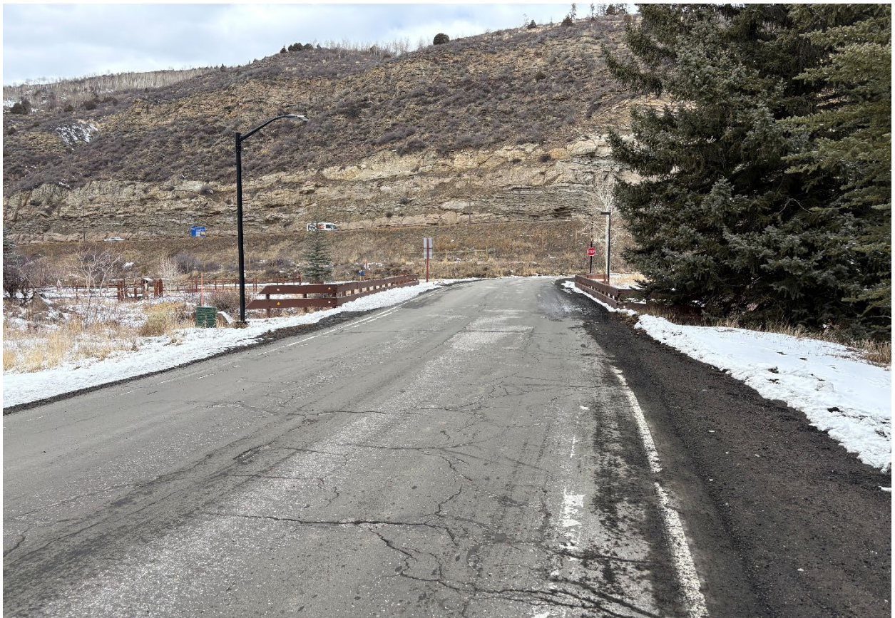
Existing condition of E. Kinnickinnick Bridge looking north.
