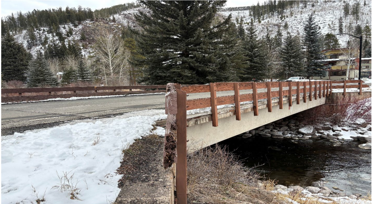
West side of the east Kinnickinnick Bridge looking south
