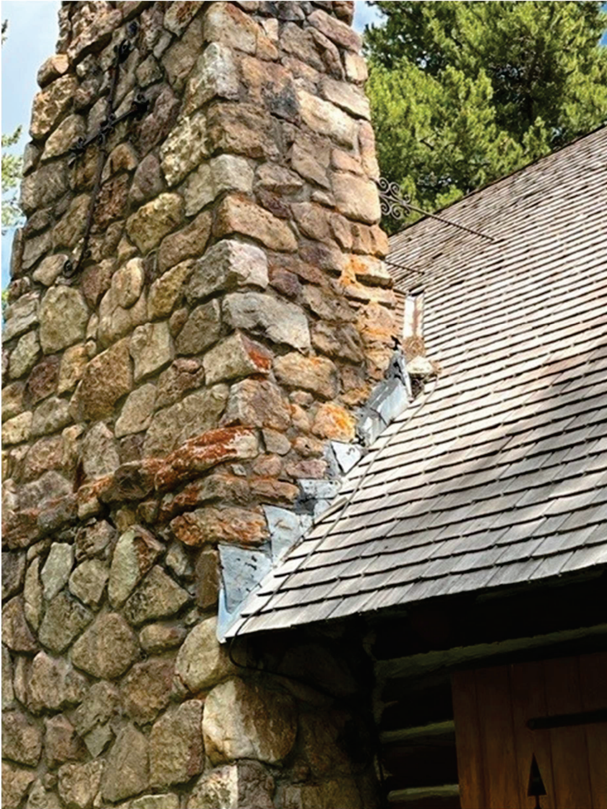
East Chimney Flashing and Masonry
