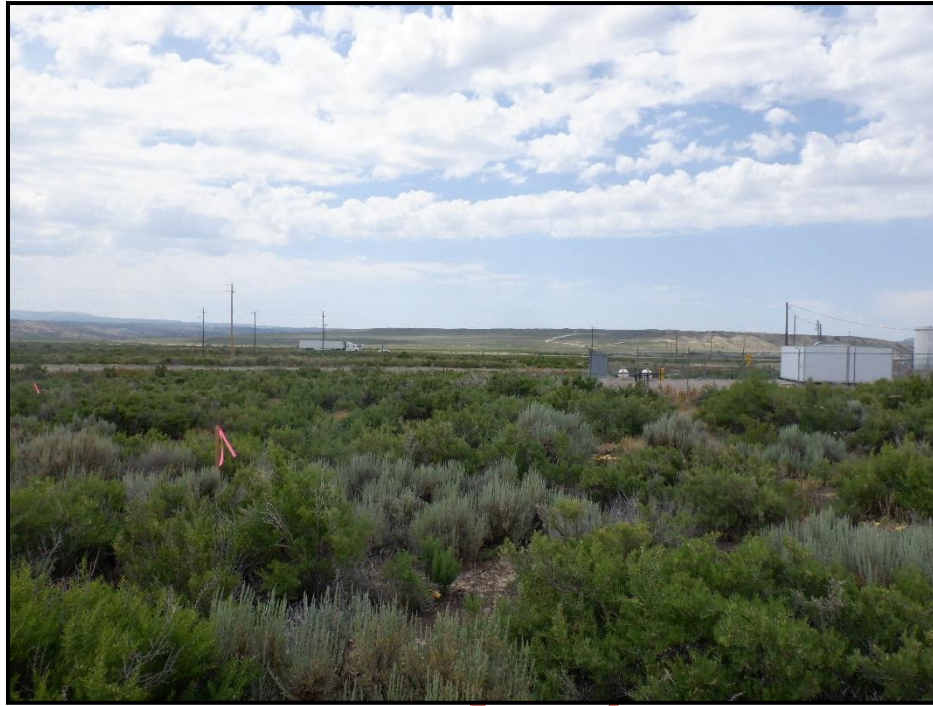
Figure 13. Overview photo of the built environment facing south from the booster station. The picture was taken by Robert Ficenec on July 7, 2022 and has not been modified.
