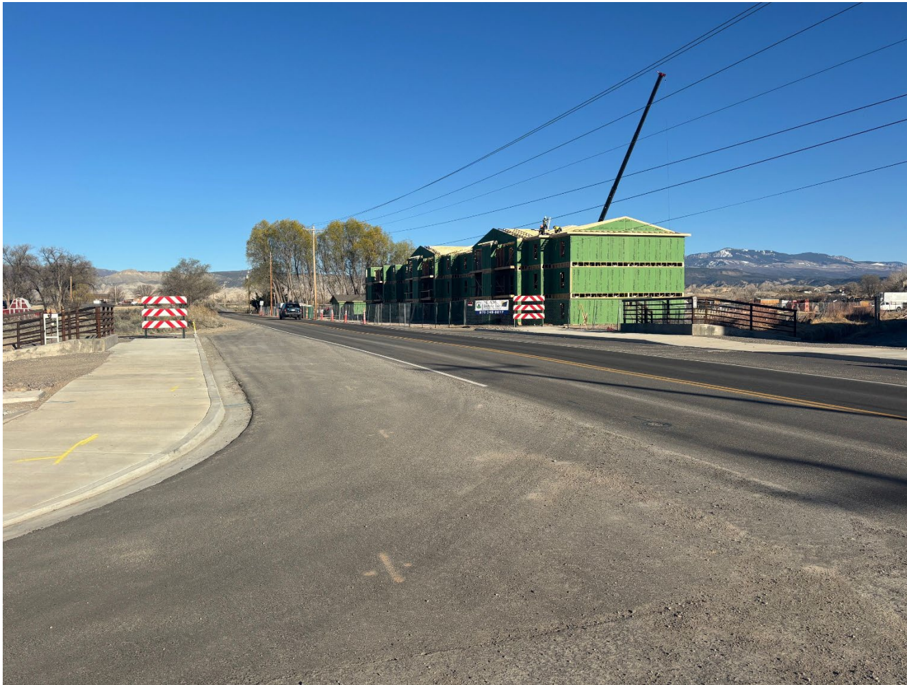
Photo 1: Completed Ogden Road Bridge
