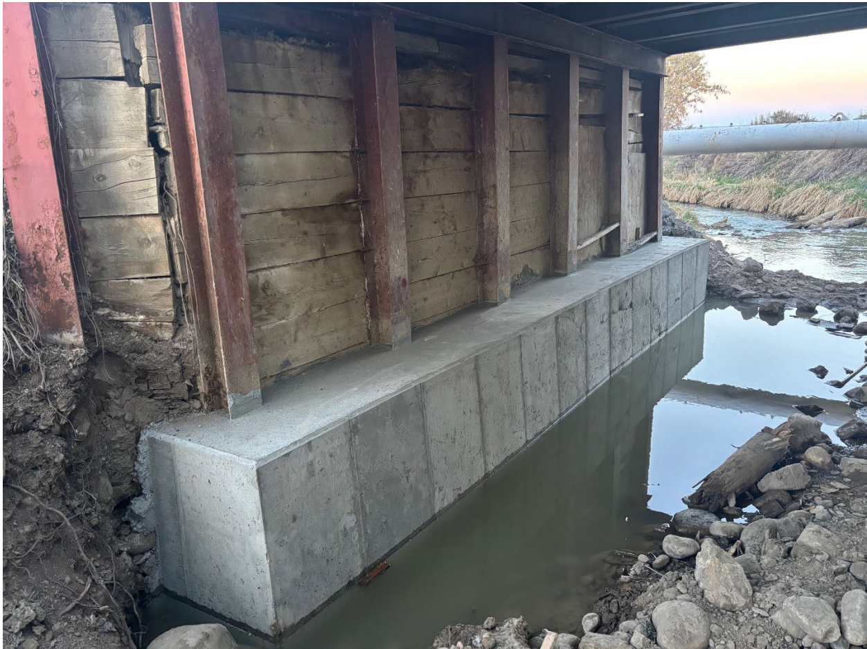
Photo 1: Completed Emergency Repair of Southern Abutment
