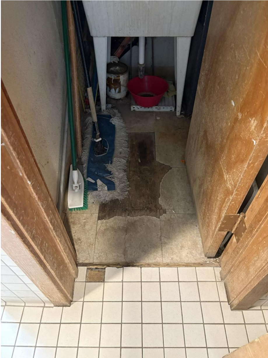
5. Miramonte 3 rd Floor tile replacement in janitor's closet.
