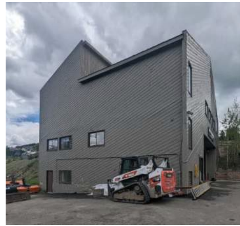
Photo #8 North elevation of the Maintenance Building
