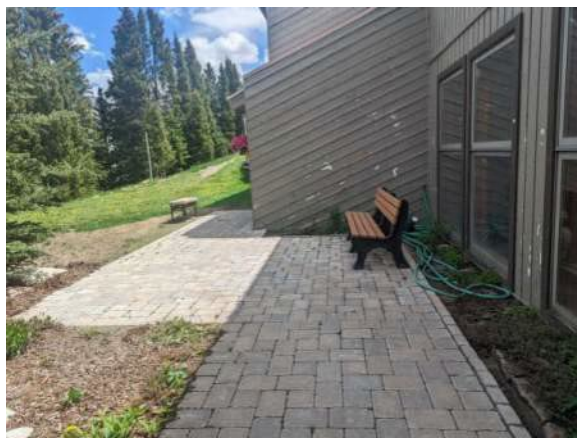
Photo #5 Western part of the South elevation Town Hall Building
