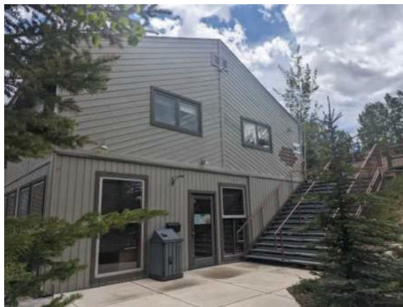
Photo #3 West elevation of the Town Hall Building
