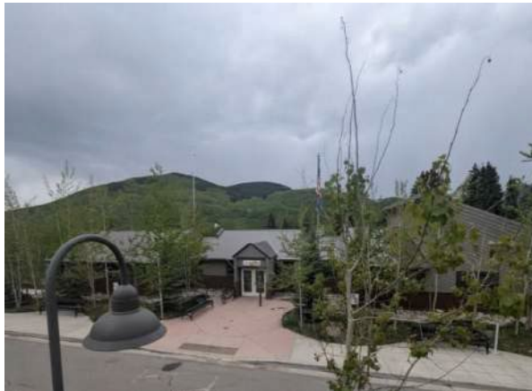
Photo #1 Front (south) elevation of the Town Hall Building
