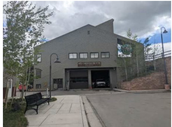
Photo #2 Front (west) elevation of the Maintenance Building
