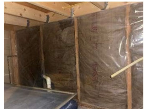
Photo 14 (above): Interior view of exterior wall assembly, with R-19 batt insulation, with some darkened/separated facer material.
