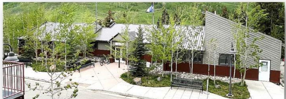
Photo 1: Overview, from adjacent Gothic Road, of the Town Hall Building in Mt. Crested Butte, CO.
