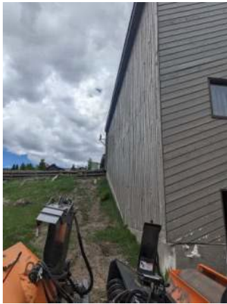
Photo #9 East elevation of the Maintenance Building
