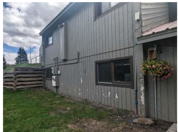
Photo #6 Middle part of the South elevation – Town Hall Building
