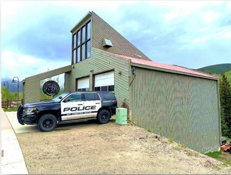
Photo 2: Overview, looking south along Gothic Road, of the Town Maintenance Facility in Mt. Crested Butte, CO.
