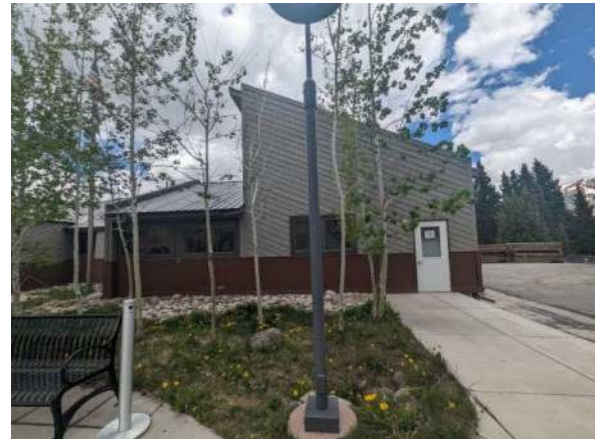
Photo #4 East elevation of the Town Hall Building
