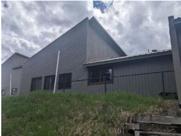
Photo #7 Eastern part of the South Elevation – Town Hall Building
