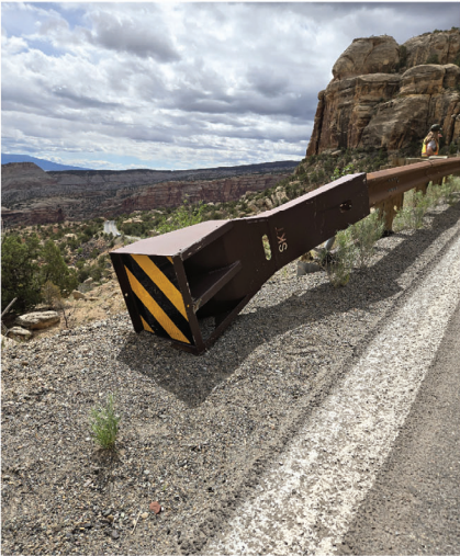
Existing Terminal Section Conditions
