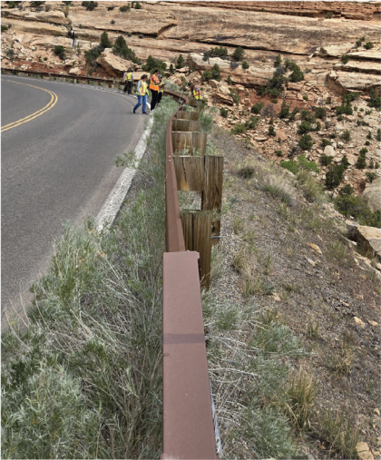
Existing Guardrail Conditions
