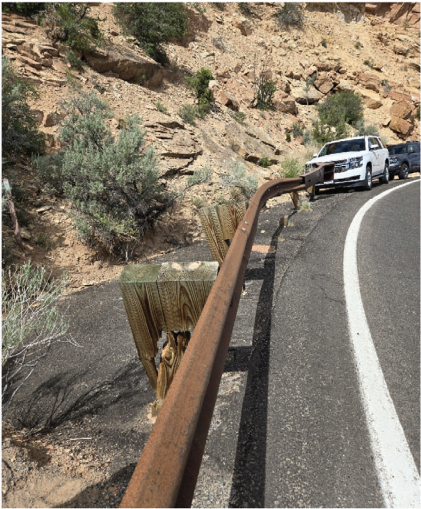
Existing Terminal Section Conditions
