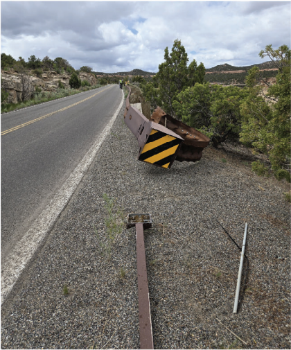
Existing Terminal Section Conditions
