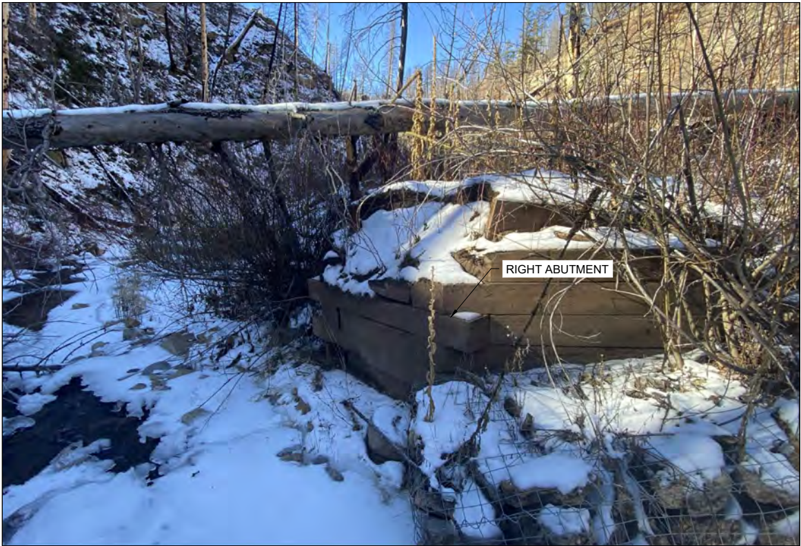
4 C-01 RIGHT ABUTMENT WING-WALL AND GABION BASKET
