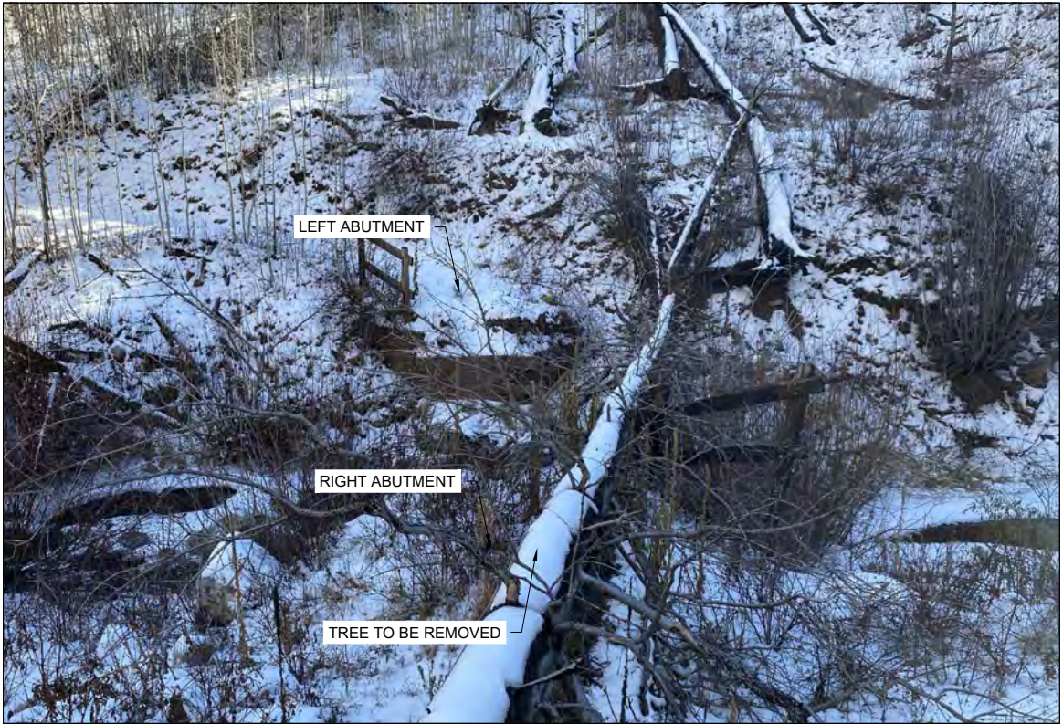
2 C-01 VIEW OF LEFT ABUTMENT AND SURROUNDINGS FROM RIGHT SIDE OF STREAM
