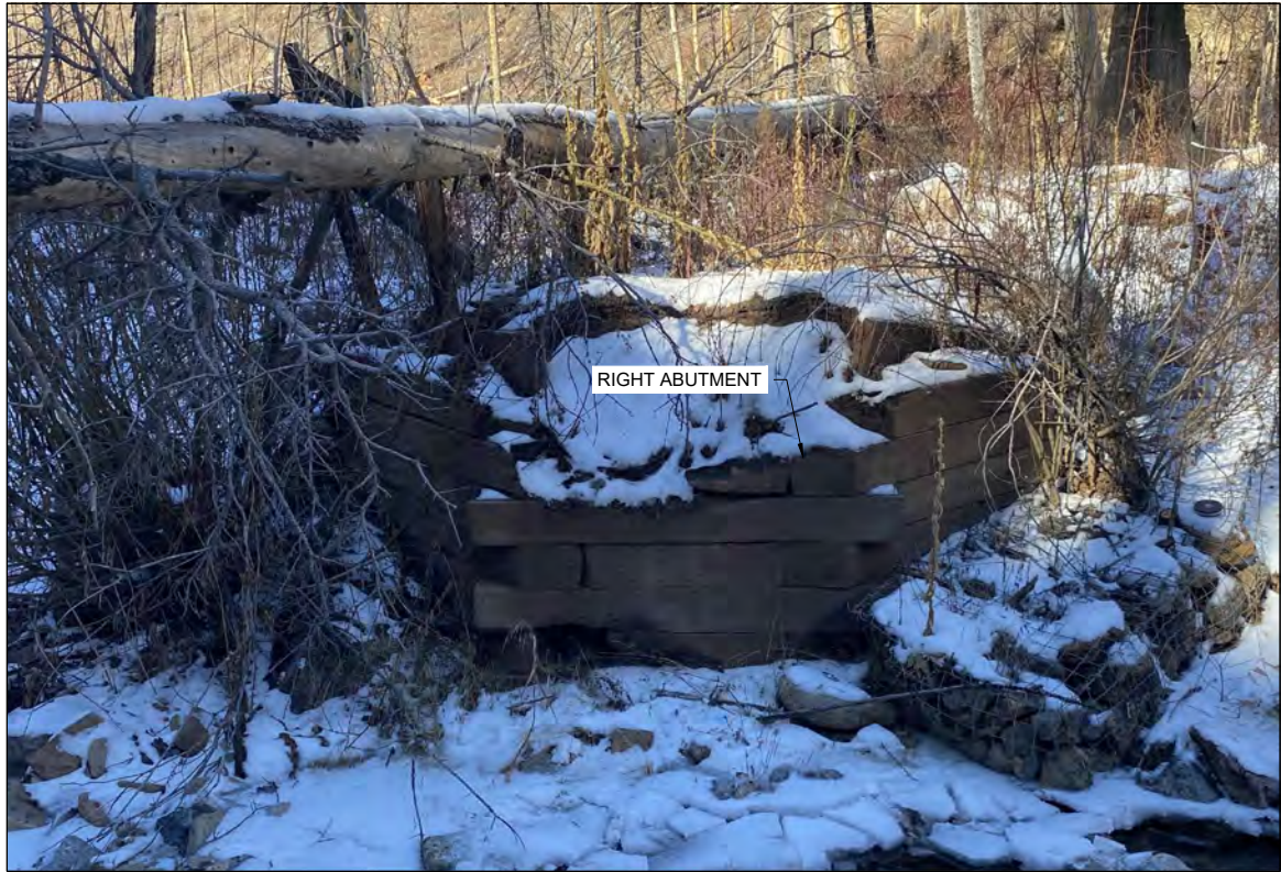
5 C-01 CLOSE UP OF RIGHT ABUTMENT TO BE FULLY REPLACED
