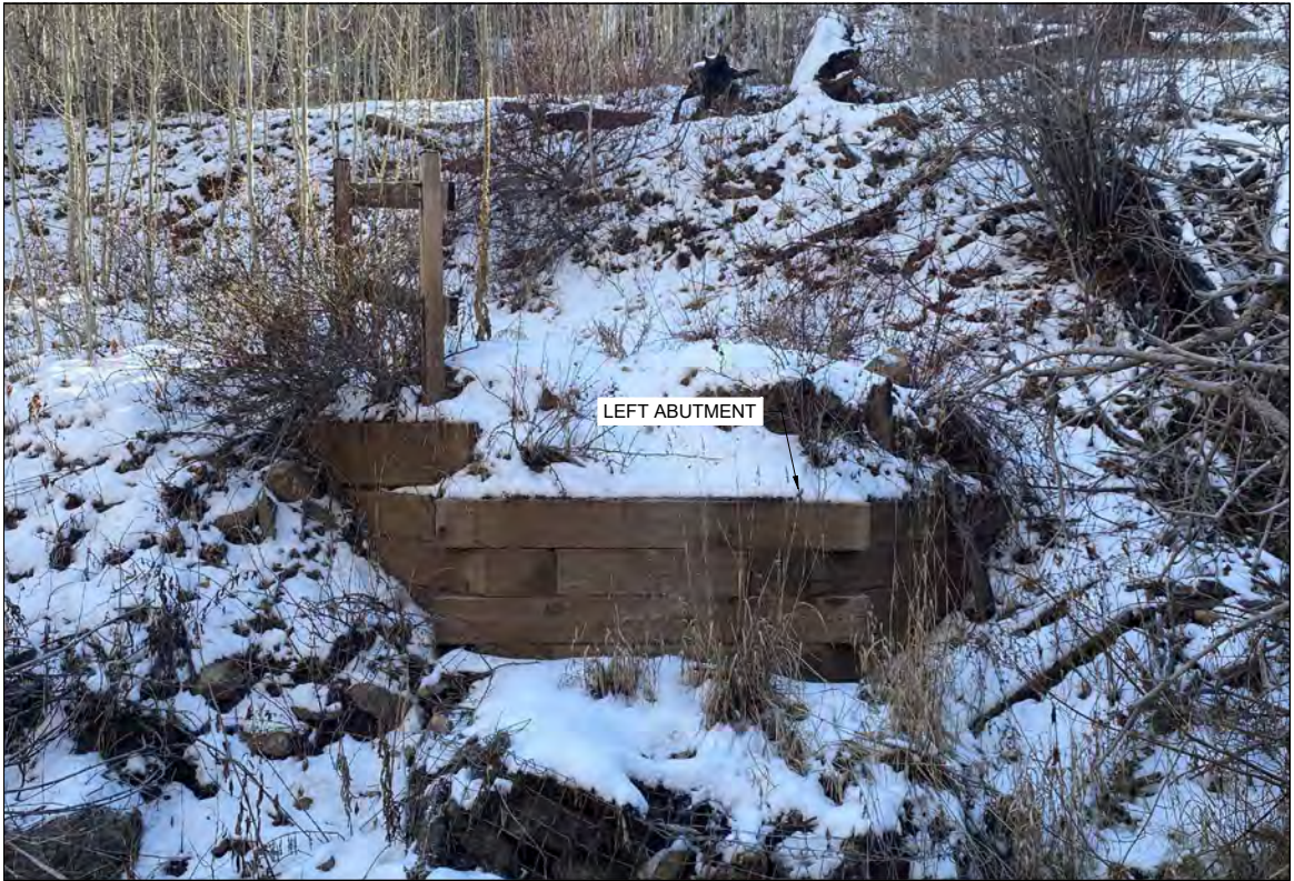
6 C-01 CLOSE UP OF LEFT ABUTMENT TO BE MODIFIED
