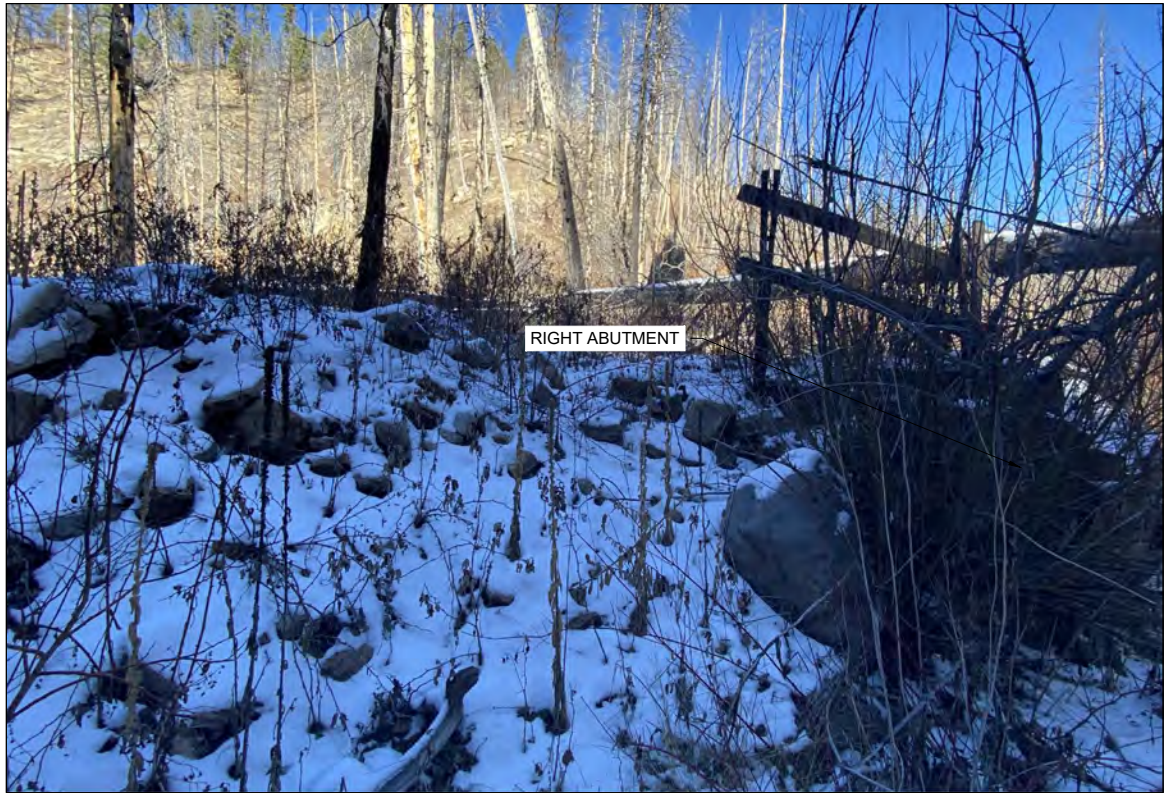
7 C-01 DOWNSTREAM SIDE OF RIGHT ABUTMENT
