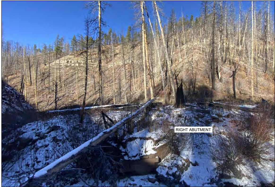
1 C-01 VIEW OF RIGHT ABUTMENT AND SURROUNDINGS FROM LEFT SIDE OF STREAM
