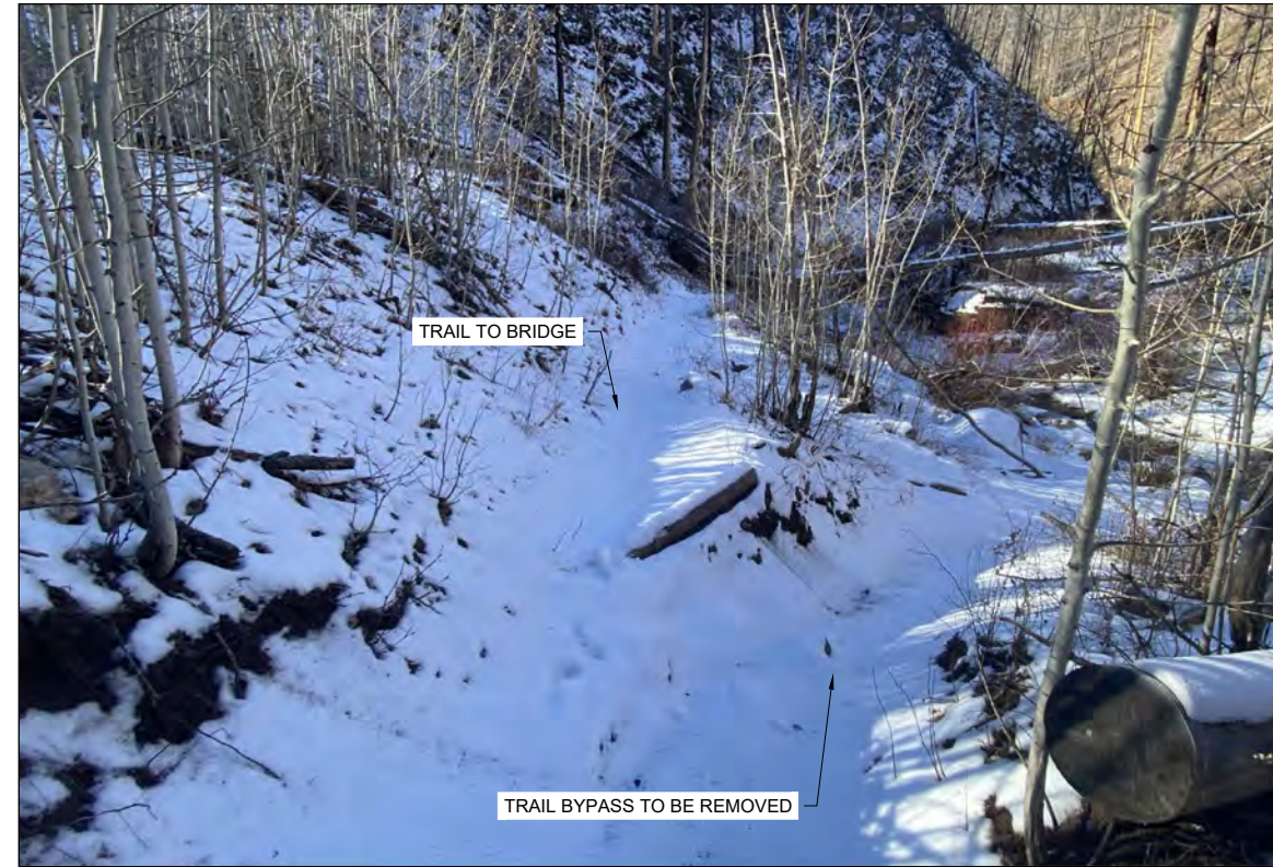
8 C-01 TRAIL APPROACH TO LEFT ABUTMENT SHOWING CURRENT BYPASS
