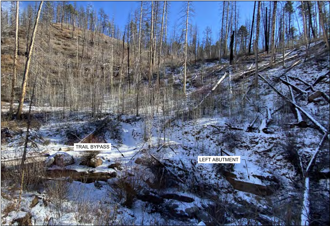
9 C-01 LEFT BANK / SLOPE
